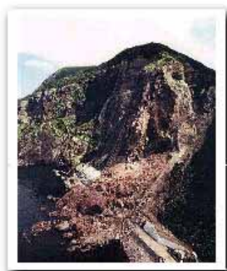
The Second Shiraito Tunnel accident
